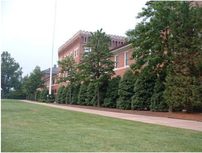
Barracks within the Marine Barracks
